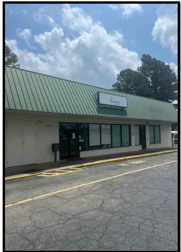
Upper School Building
